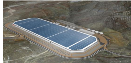
Gigafactory Feasibility Study - To assess the feasibility of establishing a UK based, scalable battery cell manufacturing facility, with the capability to ramp up to a Gigawatt hour worth of cell production
